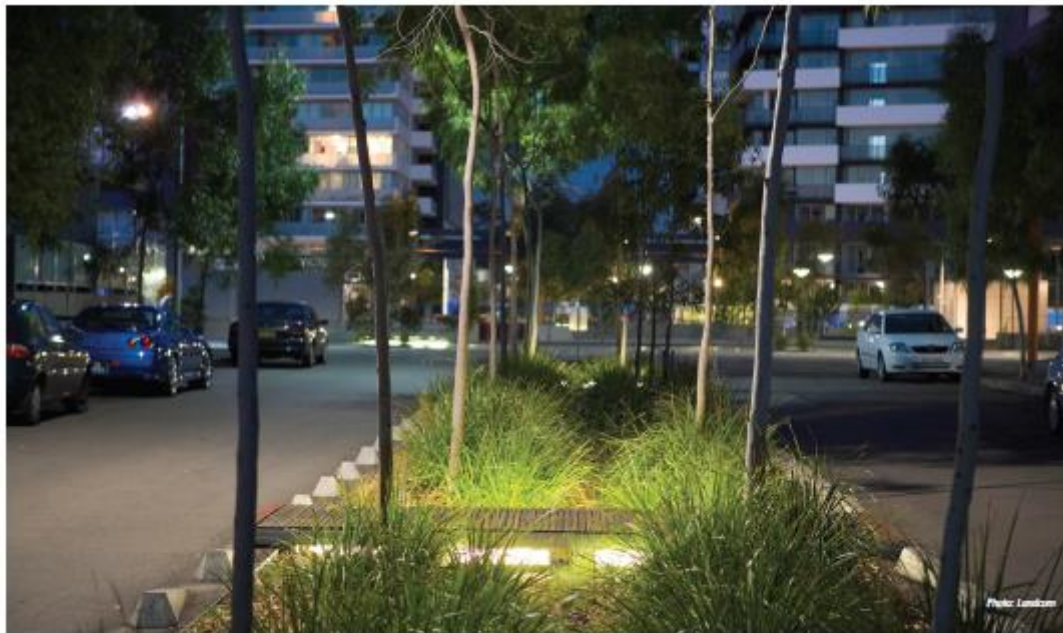
Example of WSUD street layout 4: Bioretention swale in centre median
