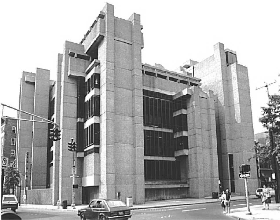
Art and Architecture Building - Yale University - Paul Rudolph (1958)
