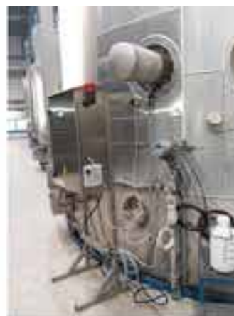
MCC too high above the seeding level
